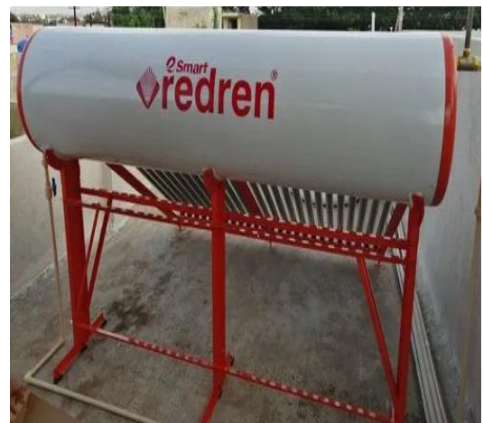
Solar Water Heater
